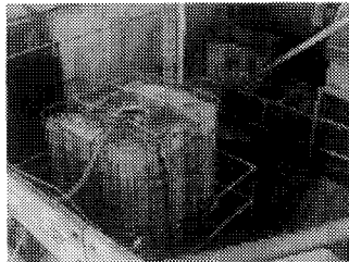
Figure 3. Picture of first grease trap
